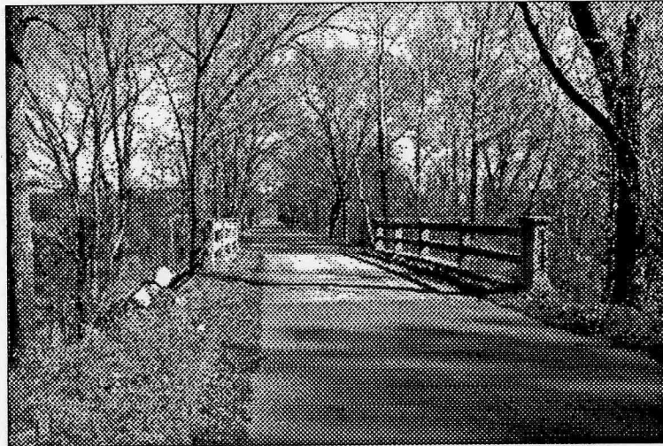
Figure D-9: Located south of Calhoun, Georgia on a bypassed alignment of the Dixie Highway's Eastern Division near U.S. 41 is this ca. 1924 T-Beam Bridge. Because it is one of fewer than 60 known T-bridges, the structure has been determined to be individually eligible for the National Register of Historic Places (photograph by author).
