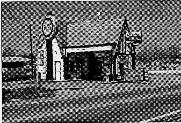
Figure D-10: Located north of downtown Cartersville is this ca. 1930 Pure Oil Gas Station, which still functions as a Pure Oil franchise (photograph by author).
