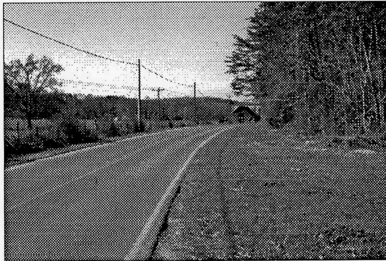
Figure B-3: A large part of the Dixie Highway's Western Division through North Georgia is found on present-day U.S. 27. However, in several places, the numbered route lies on a new alignment that has bypassed the old road. This photograph shows a section of the former alignment in rural Walker County, Georgia (photograph by author).
