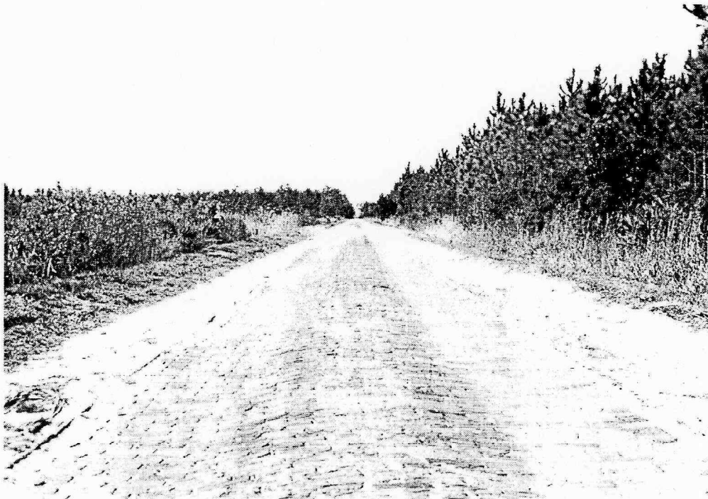
Figure A-30: Brick paved section of the Dixie Highway, Flagler County, Florida
